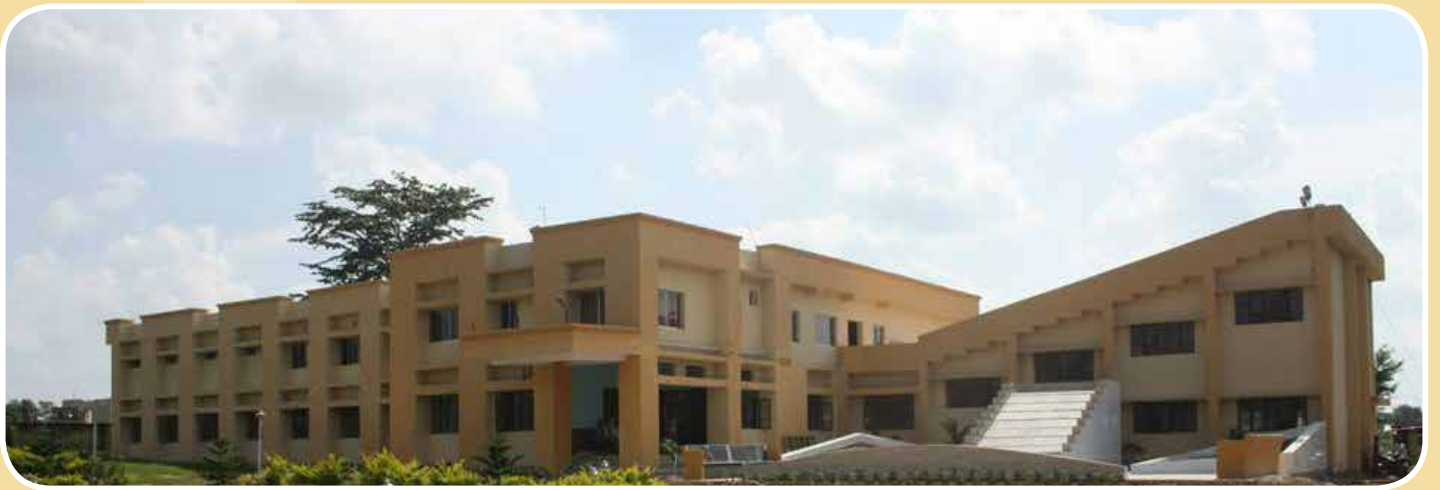
Well furnished Wi-Fi Building
